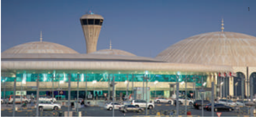
1 AIR CONTROL TRAFFIC TOWER AT SIA
